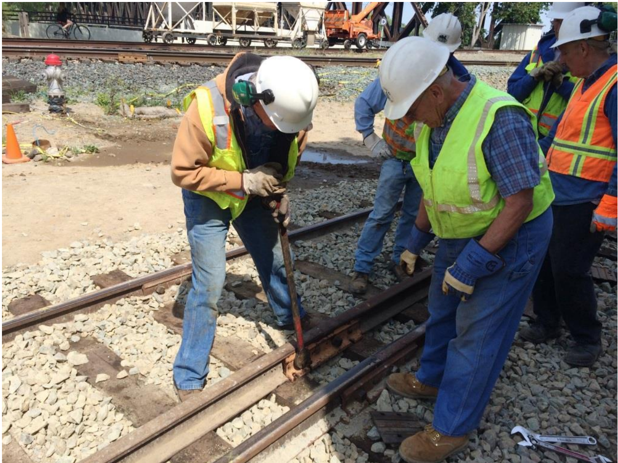
Steve and Clem join the two rails and bolt them in place
